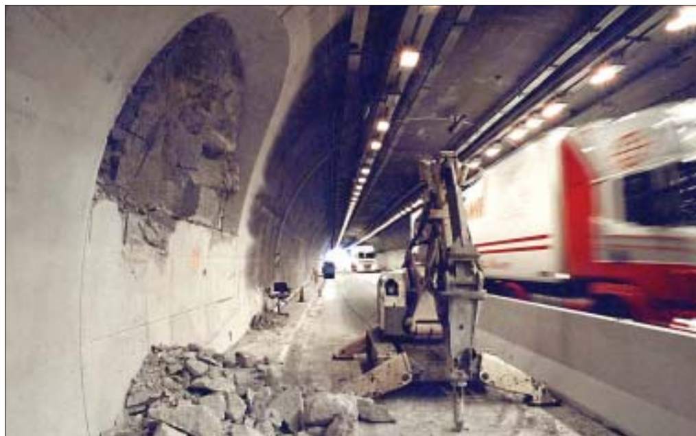
Fig 4 (above) Concrete being jack-hammered away to form the alcove
